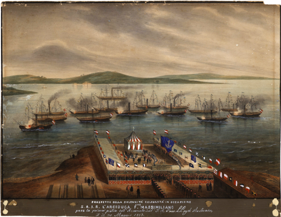
FIGURE 15.2 Celebrations for the laying of the foundation stone of Austrian Lloyd's shipyard (30 May 1853)
